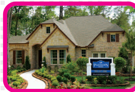
Plantation Homes in Overland Trace
